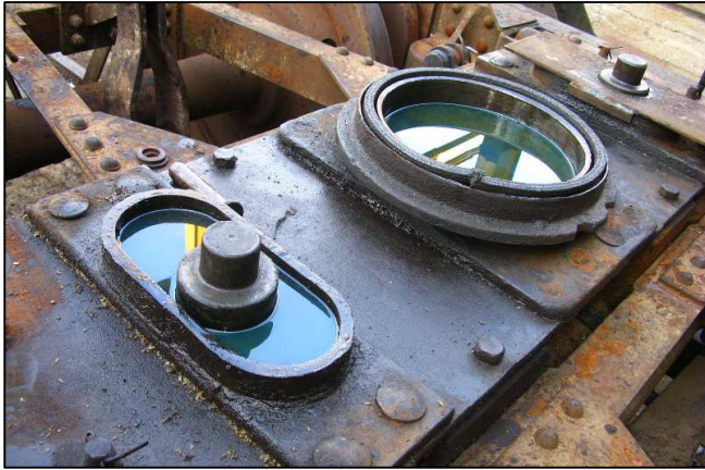
P03 - The newly repaired boss now holds oil as designed. Square-section graphite packing was installed as a seal.
