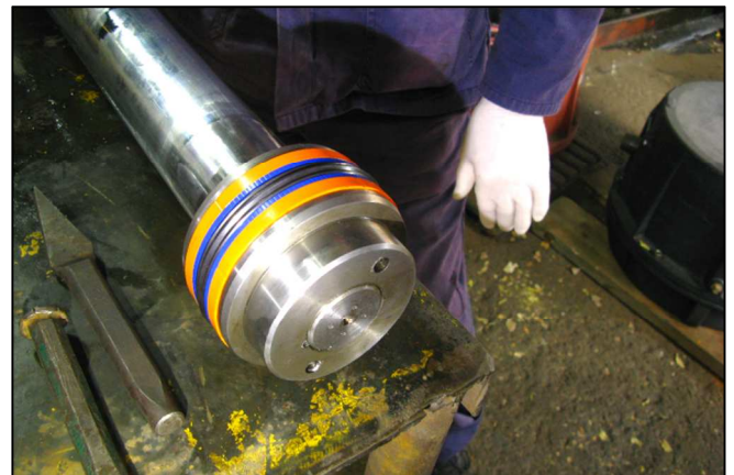
P08 - Brightly coloured hydraulic seals and spacer rings being installed for the extension boom of the coal grab.
